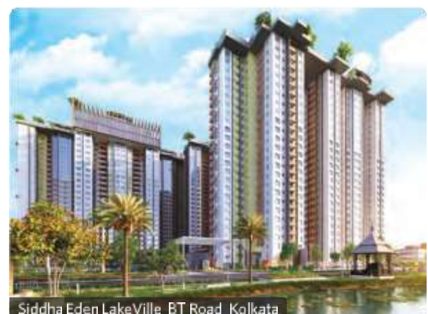
Siddha Eden LakeVille BT Road Kolkata North Kolkata's first Rooftop Skywalk Phase 1 - HIRA/P/NOR/2018/000183 | hira.wb.gov.in Phase 2 - HIRA/P/NOR/2019/000385 | hira.wb.gov.in
